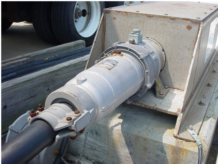
Figure 13-2. Close-Up of Electrical Connection Outlet Assembly
