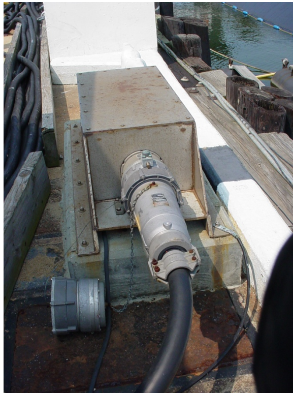
Figure 13-2. Close-Up of Electrical Connection Outlet Assembly
