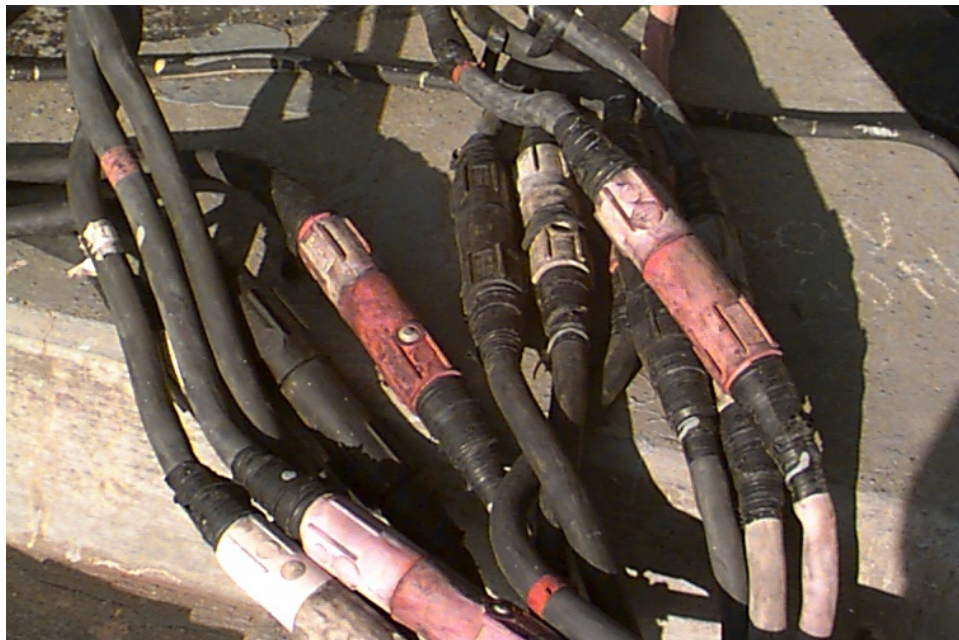
Figure 13-11. 480 Volt Shore-Cable to Ship-Cable with Single-Pole Connection
