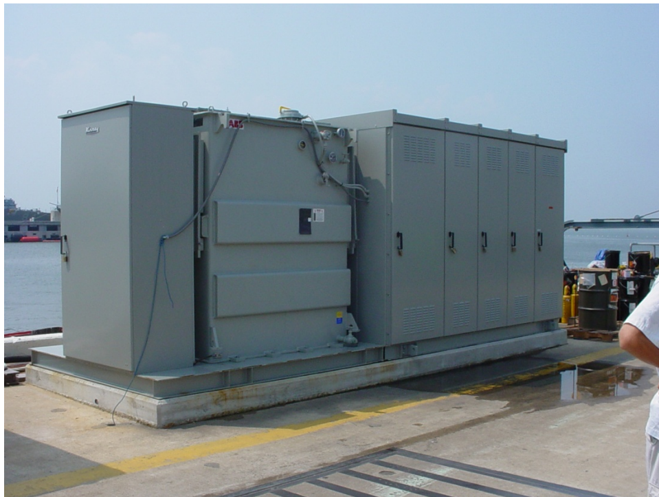
Figure 13-4. Skid-Mounted Substation
