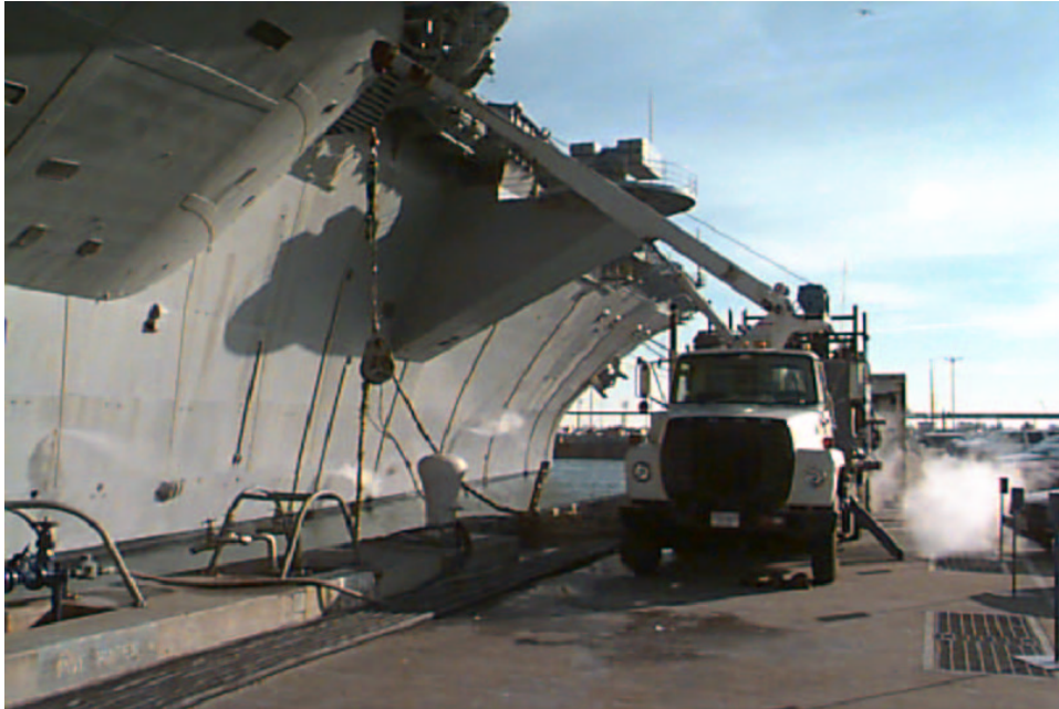
Figure 13-17. Cable Being Reeled by a Boom Truck.
