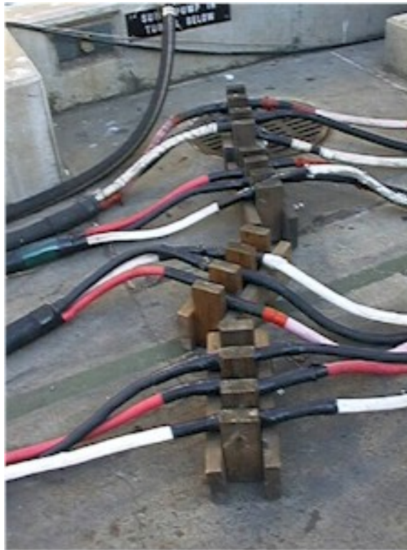
Figure 13-13. 480 Volt Shore-Cable to Ship-Cable Splice Connection in Place
