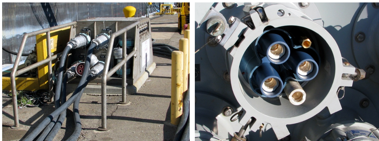
\2\ Figure 13-9. 4.16 kV Pier Electrical Outlet Assembly and Outlets – Newer Designs
