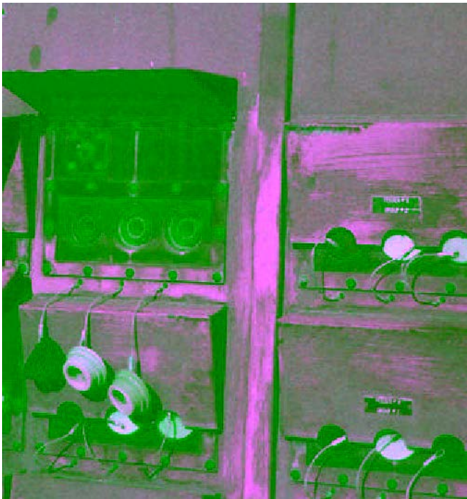
Figure 13-6. Newer Double-Deck Pier Switchgear
