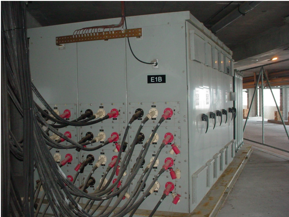
Figure 13-6. Newer Double-Deck Pier Switchgear
