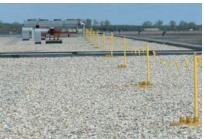
Fig. 7: Warning lines keep workers aware of and away from roof edges.
