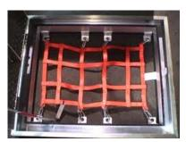
Fig. 8: Net coverings prevent workers from falling to lower level.
