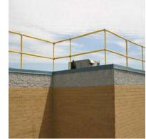
Fig. 1: Guardrails along roof edge
